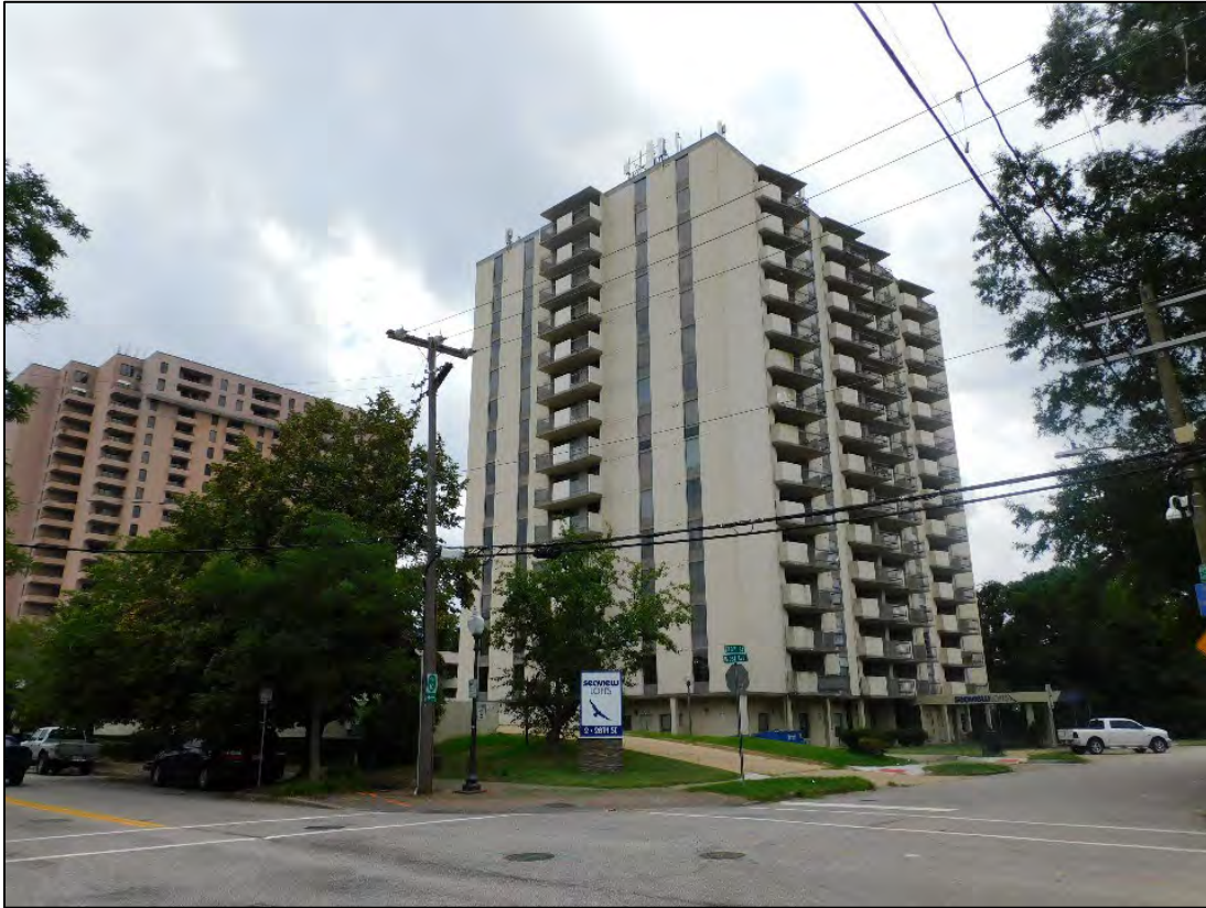
Figure 6: 90 28th Street, Seaview Lofts (DHR# 121-5621-0029)
