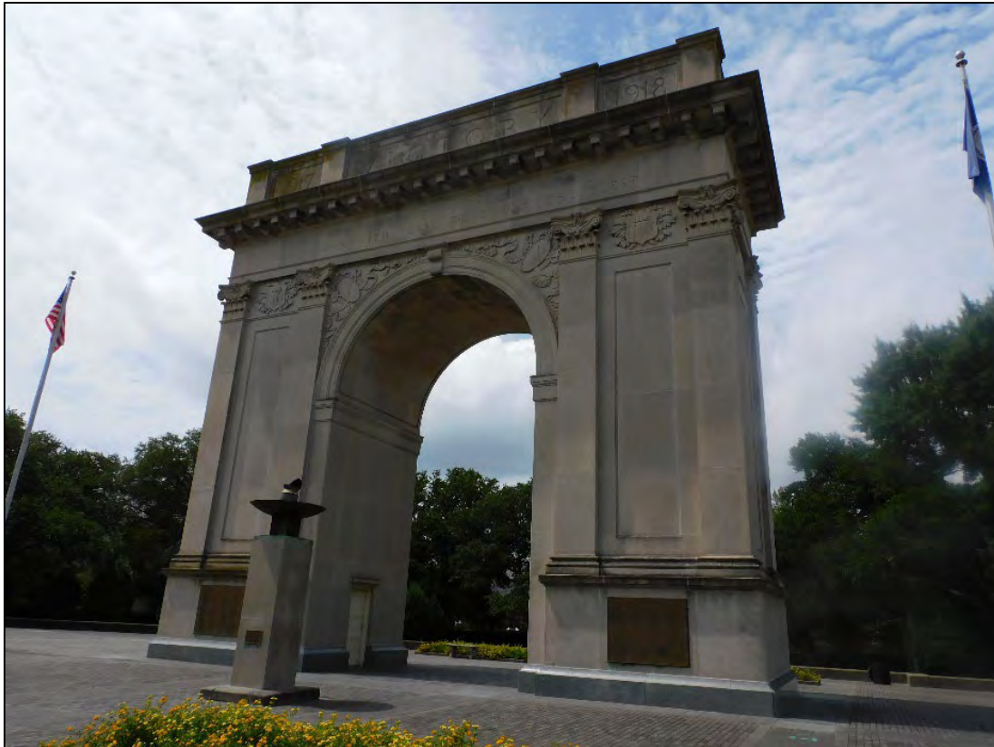
Figure 12: 2501 West Avenue, Victory Arch (DHR# 121-5621-0058)
