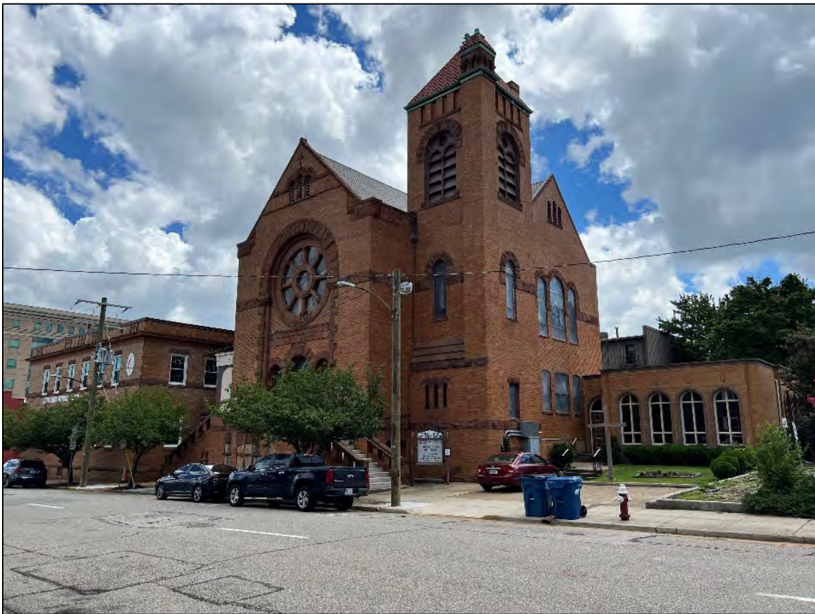
Figure 10: 228 29th Street, Trinity United Methodist Church (DHR# 121-5621-0057)
