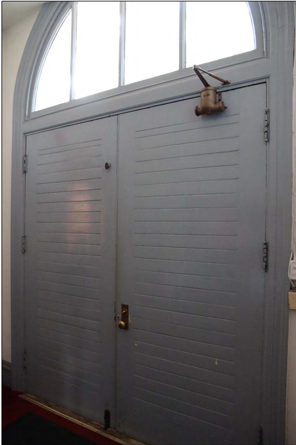
PHOTO 21: View of Main Entrance Doors from Inside Vestibule (N. Holst, August 29, 2022)
