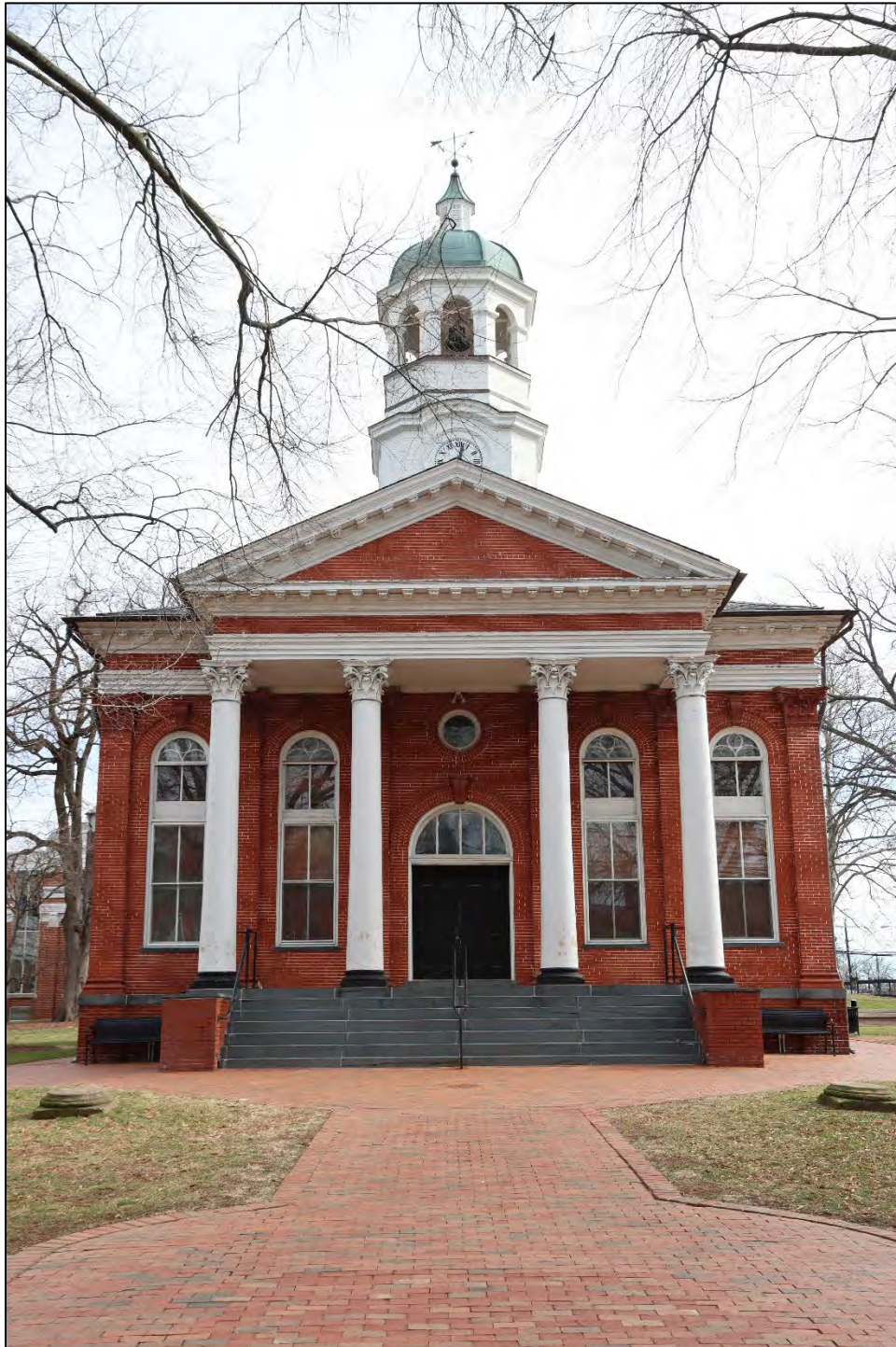
PHOTO 4: View Southeast Toward Main Façade, Loudoun County Courthouse (N. Holst, January 28, 2023)
