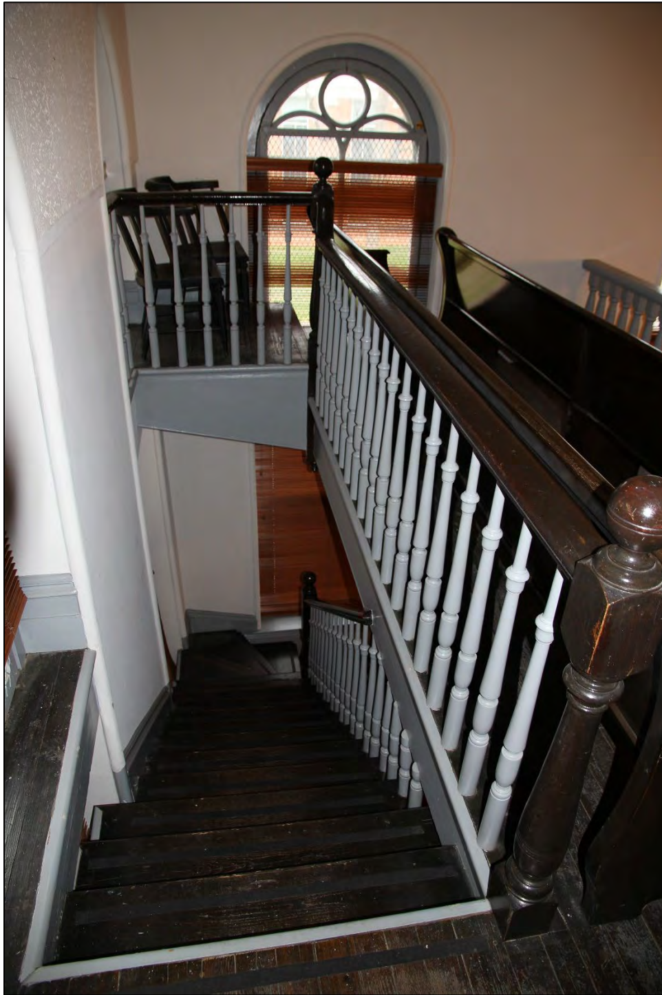
PHOTO 19: View of Stairway from Gallery (N. Holst, March 24, 2022)
