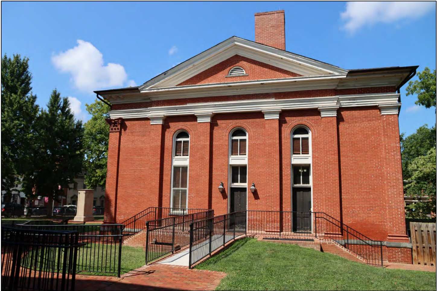
PHOTO 13: View Toward Rear (southeast) Façade of Loudoun County Courthouse Showing Original Rear Entrance Used in the 1933 Trial (center) and Second Rear Entrance (right) Installed at a later date (N. Holst, August 29, 2022)
