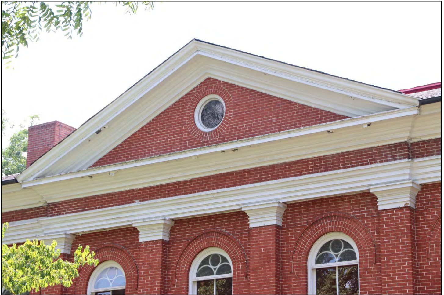
PHOTO 7: View of Cross-Gable Pediment, Northeast Façade (N. Holst, August 29, 2022)
