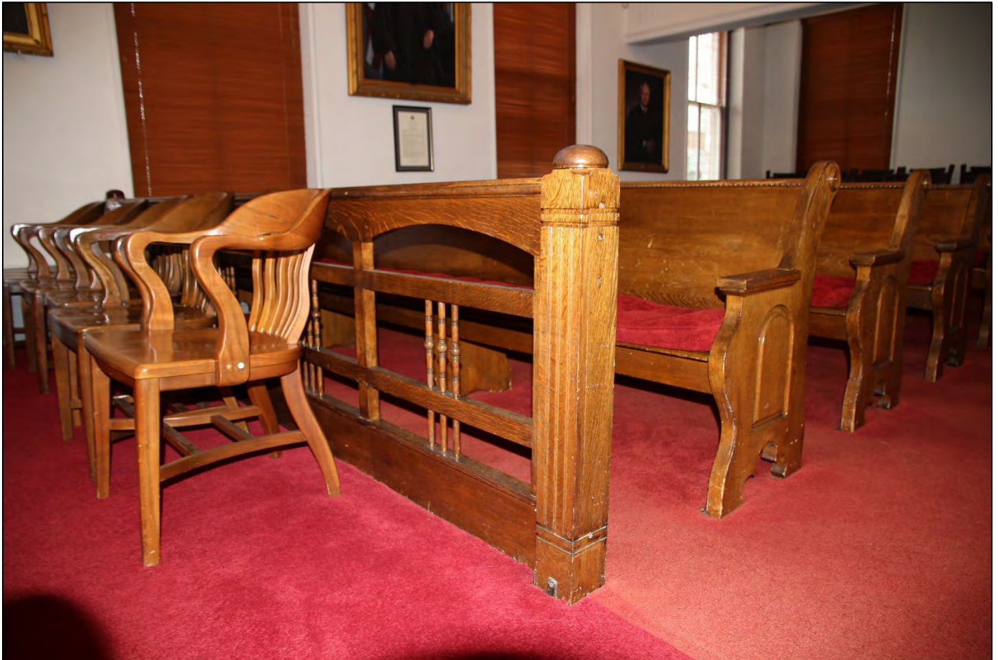
PHOTO 24: View of Historic Railing (bar) and Spectator Benches Present in 1933 (N. Holst, March 24, 2022)
